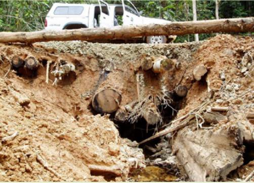
*Excessively cleared and poorly constructed roads and bridges have major impacts on environmental values and often fail, causing disruption to haulage systems and necessitating high maintenance and repair costs.*
